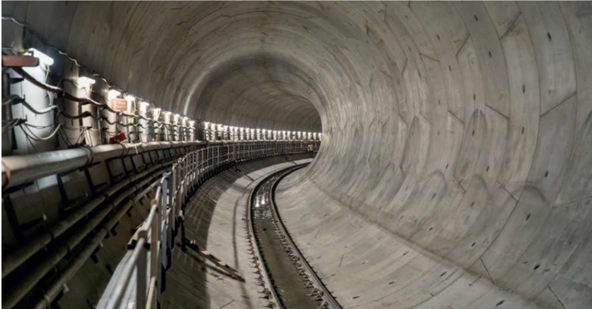
The tunnel structure was created without the need for left- and right-hand segments PHOTO: ABSOLUTE PHOTOGRAPHY LTD
